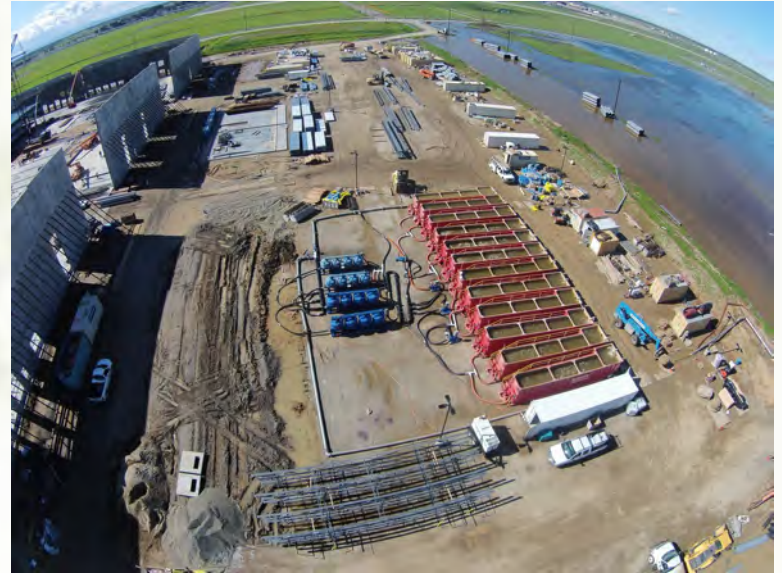
With 20 years of experience, ATS has the experience to get the job done right! Pictured: 2,800 GPM ATS
